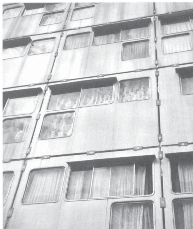
Fig. 5. Blanc Mesnil, elevation with “clip-on” panels by Jean Prouvé, 1956.
